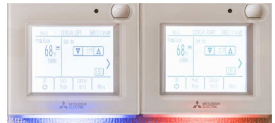
Inside Minnesota Power’s conference room, two side-by-side thermostats, each connected to a different indoor unit, light up with blue to indicate cooling or red to indicate heating. The utility company uses the thermostats to explain simultaneous heating and cooling.
